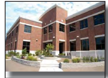
^ The newly completed Horton Building
